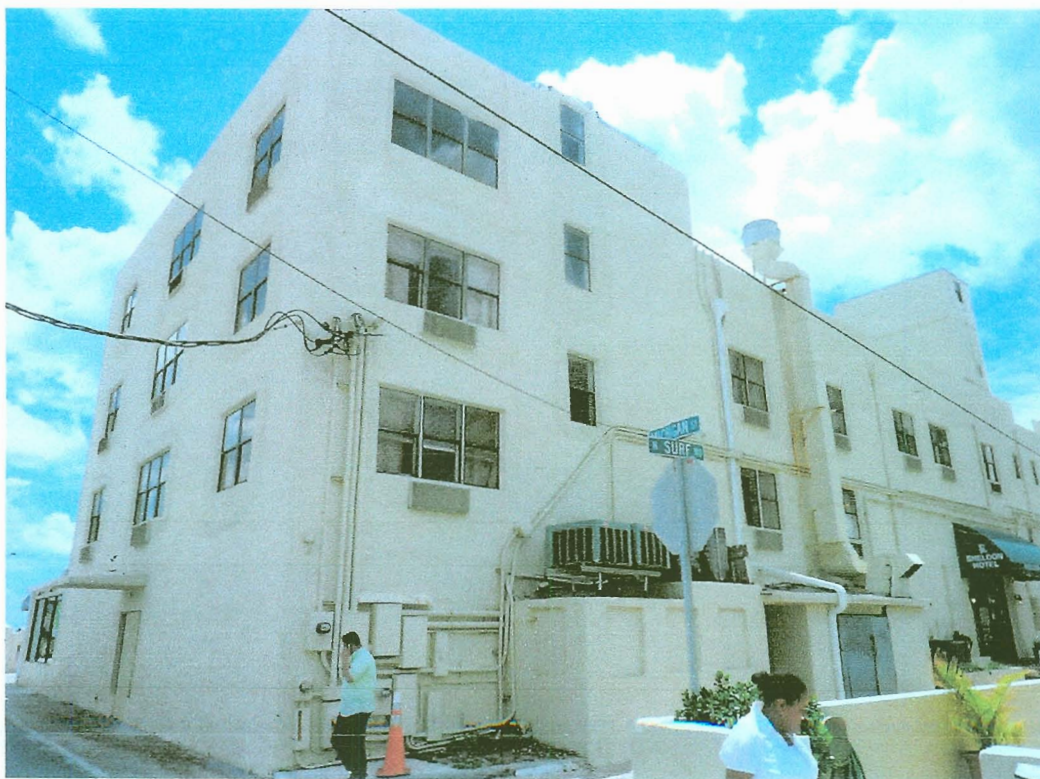
EXISTING NORTHWEST VIEW
